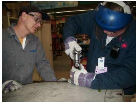
Figure 6: Bill Tate (right) shows new hand Murray Beaulieu how to remove old rivets
